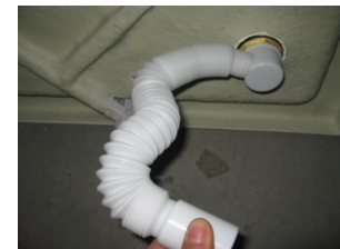
DRAW PIPE TO DRAINAGE HOLE.
