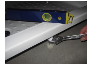
MAKE TRAY LEVEL BY ADJUSTING SCREWS.
