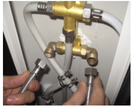
CONNECT HOT&COLD PIPE
