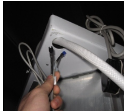
ELECTRIC LINES THROUGH THE HOLE
