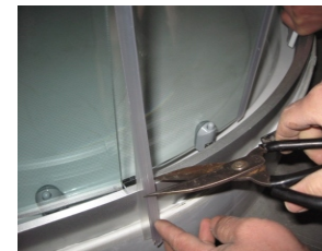
INSERT WATER PROOF TYPE&CUT OVERAGE
