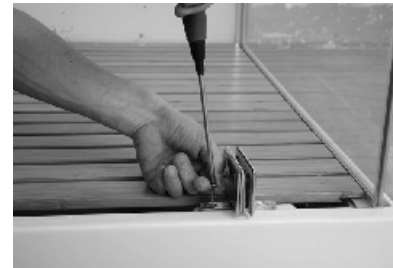
33. Fix the joint scrow of hinge and tray .
