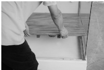
29. Install the bamboo floor.
