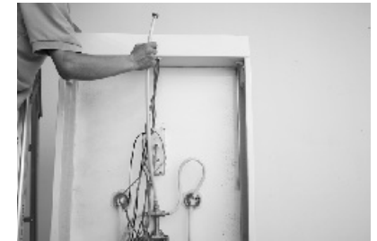
46. Make the inlet pipe going through the drilled hole of roof.
