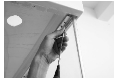
21. Install the joint screw of roof and side panel.
