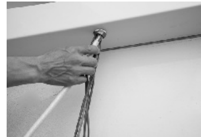
45. Be ready to install the inlet pipe of top shower.
