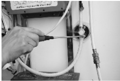
49. Fix the screw of clip as the picture.
