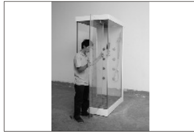
38. Install the movable glass door.
