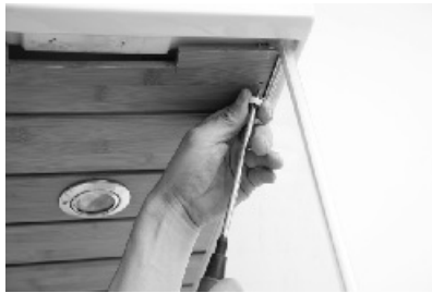
25. Install the joint scrow of roof and bamboo roof.
