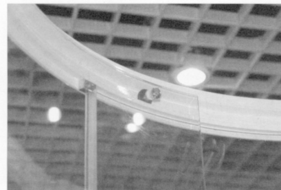
19. Lean the sliding glass, move the attached ball bearing into the track
