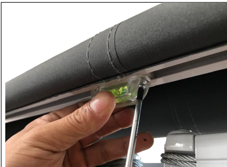
Fix the spirit level in the middle
