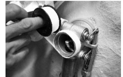
2. Use thread sealing tape to wrap around the drain hole
