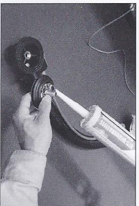
56. Seal with silica gel around the drainer as pic show and make sure no silica gel left inside of the drainer.
