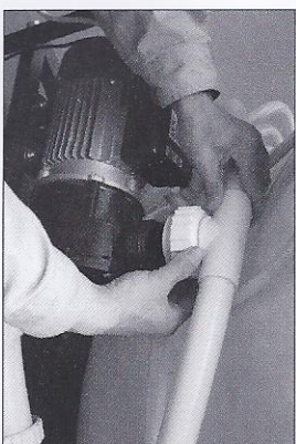
68. Connect the main water pipe to the pump.
