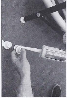
14. Seal with silica gel around the small water jet .
