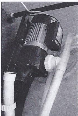
69. Tighten the main pipe to the water pump as pic shown.
