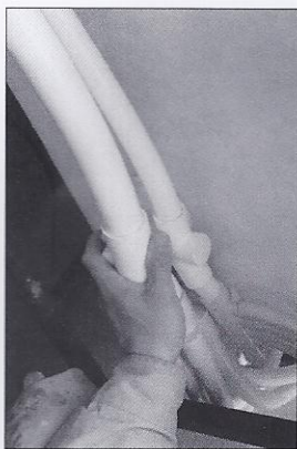
22. Fix the water pipe connector to the big water jet.
