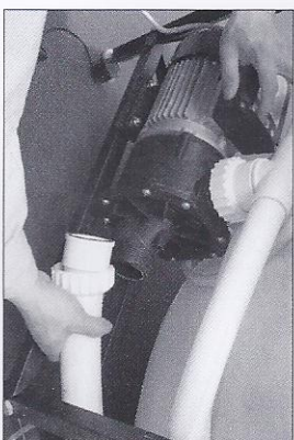
70. Connect one end of waterback pipe to the water pump.
