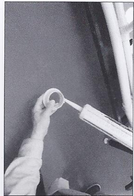
19. Loosen the big water jet and seal with silica gel around it.
