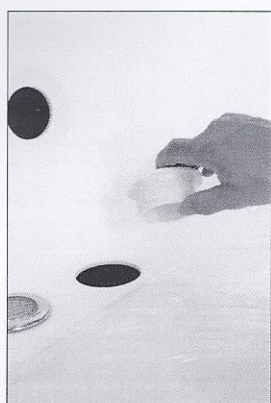
32. Insert the waterback to the hole.
