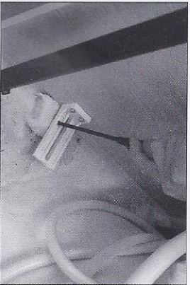
11. Tighten the screw to make sure the "L" shaped connector connects well.
