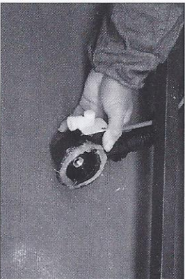
57. Insert the drainer end to the hole from back side.
