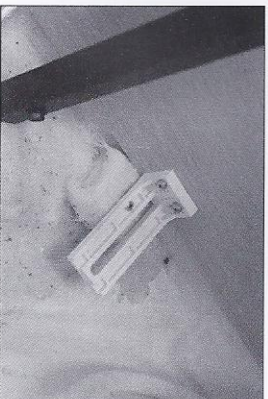
10. Fix one side of "L" shaped connector to the tub edge.
