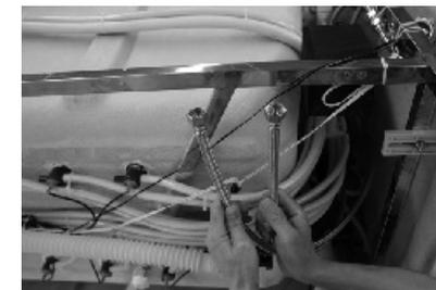
10. Connect the cold and hot water pipes .
