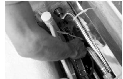
4. Put the rubber from below, and use spanner to screw it.
