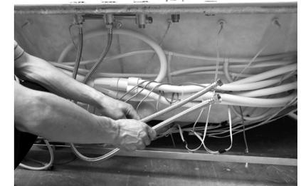
10. Connect the cold and hot water pipes .
