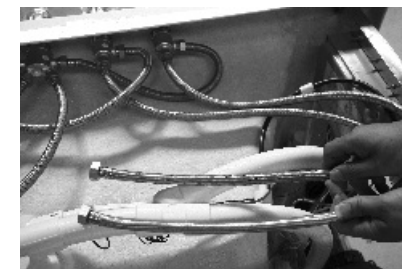
10. Drain sewage of the tube, then connect the cold and hot water pipe separately
