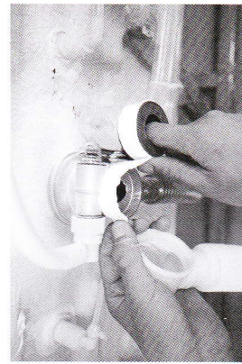
6. Use thread sealing tape to wrap around the drain hole
