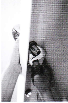
4. Put the rubber from below, and use spanner to screw it
