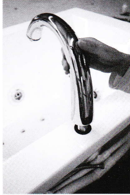
3. Put the inlet faucet into the hole of the bathtub
