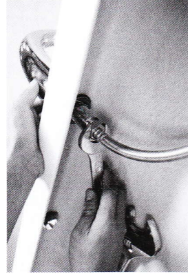
6. Use spanner to screw the tie in.
