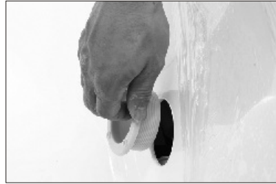
16. Insert the big water jet to the tub.
