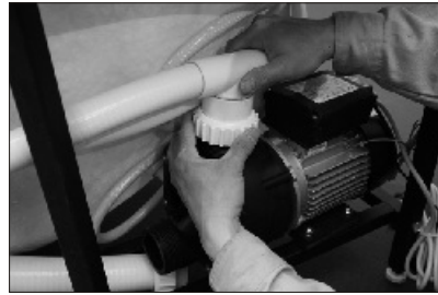
62. Connect the main water pipe to the pump.
