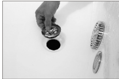
52. Put the drain cover from front side into the drainer and make sure the right direction.
