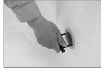
19. Tighten the big water jet with a special spanner.
