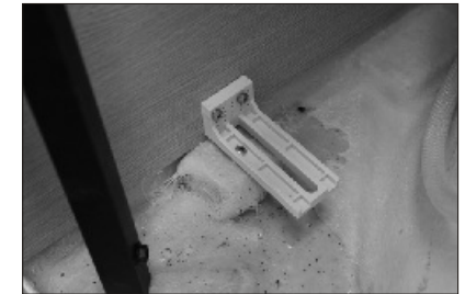
10. Fix one side of "L" shaped connector to the tub edge.
