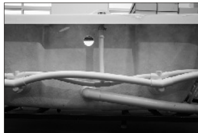
38. Make sure the pipe and button is well-connected as pic shown.
