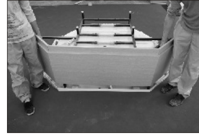
7. Put the protection foam on the floor then side up the tub, put on the whole skirt.
