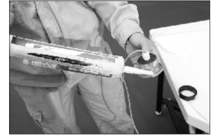
22. Seal with silica gel around the underwater light.
