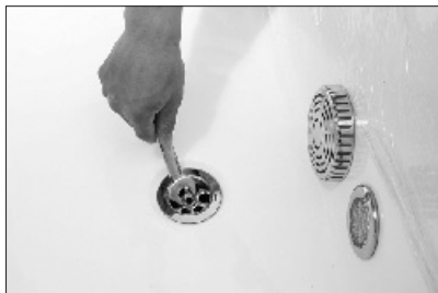
53. Tighten the screw with spanner.
