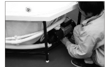
60. Fix the water pump to the frame with M6x40mm screw as pic shown.
