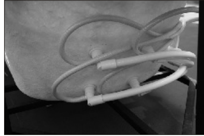
14. Connect all the small water jets to the pipe connectors.
