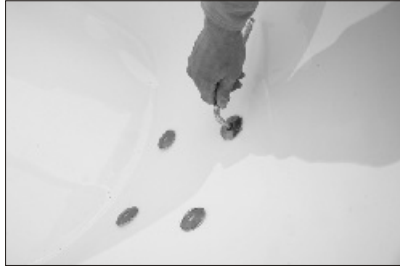
13. Tighten the small water jet with Allen key.
