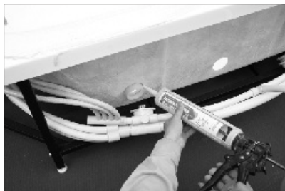
17. Seal with silica gel around the big water jet from backside.
