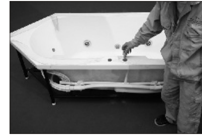
31. Loosen the screw nut of volume control button and insert it to the tub as pic shown.
