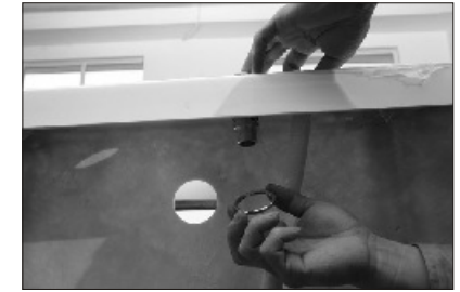
32. Tighten the screw nut as pic shown.
