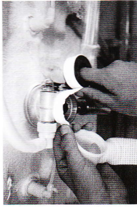
2. Use thread sealing tape to wrap around the drain hole
