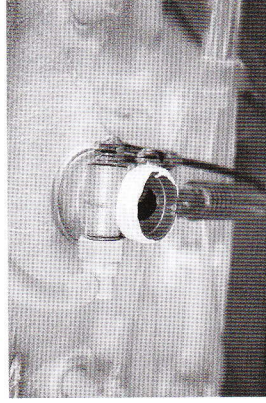
3. Make the thread sealing tape smooth
